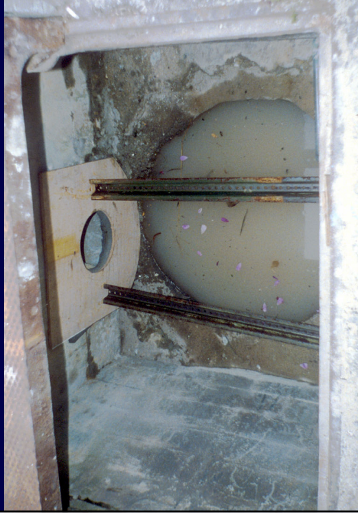
Retro-fitted Catchbasin with Sump Tested at Ocean County, NJ
